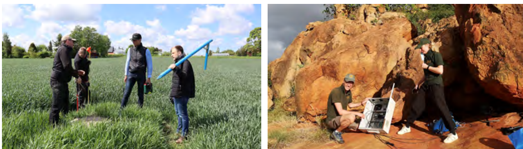
Left: Installation of sensor and communication infrastructure. Right: Fredrik Gustafsson and Sara Ohlsson installing a field station in Kenya, a system that inspired parts of the technology now applied in agriculture. Photo: Team Ngulia.
